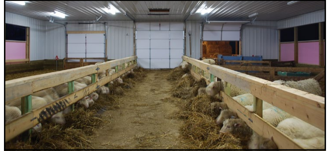
Figure 3. An insulated, indoor birth facility with a center aisle feeding system. This barn has sufficient attic insulation to stay above freezing during the vast majority of winter in southern Michigan with animal heat alone. Side wall curtain ventilation allows for air intake and exhaust. Balancing humidity and warmth requires management finesse in such a system.
